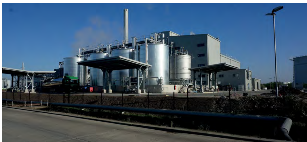
Argent's biodiesel plant
