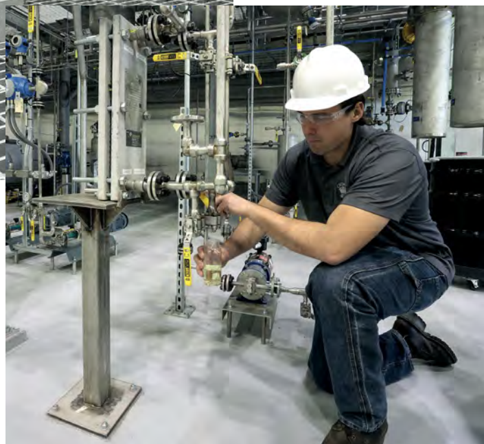
Work being carried out at the plant
